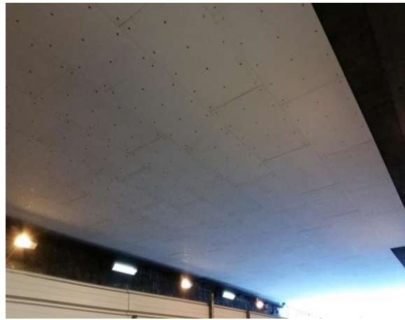
SEVINE TUNNEL, FRANCE
