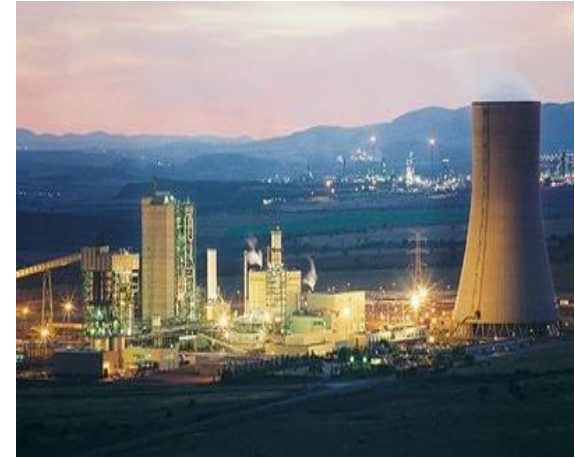
REPSOL REFINERY, SPAIN
