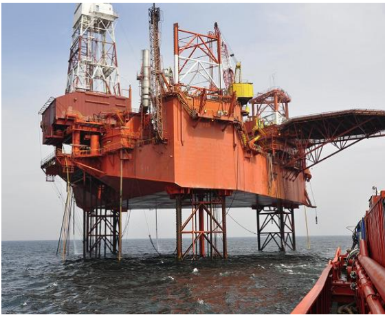
LOTOS PETROBALTIC DRILLING PLATFORM, POLAND
