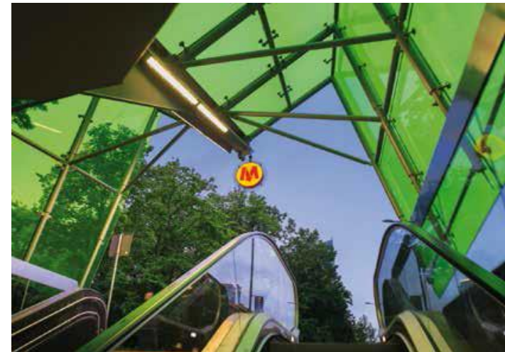
WARSAW METRO, POLAND
